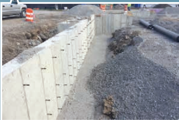
SEPT. 16, 2016 Foundation and excavation starts
