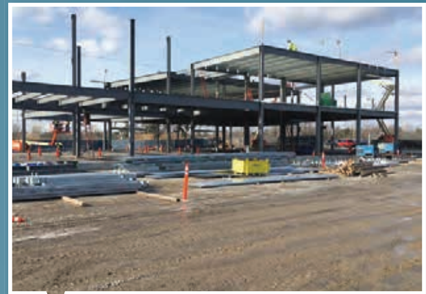
DEC. 19, 2016 Steel erection starts
