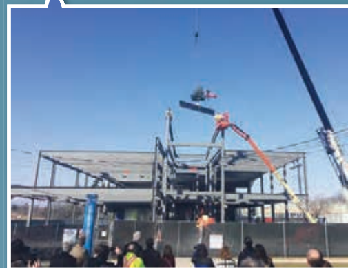
FEB. 27, 2017 Steel complete/ topping out
