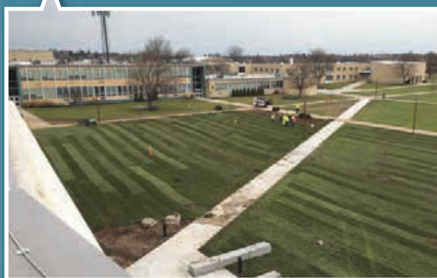
NOV. 10, 2017 Sod installation
