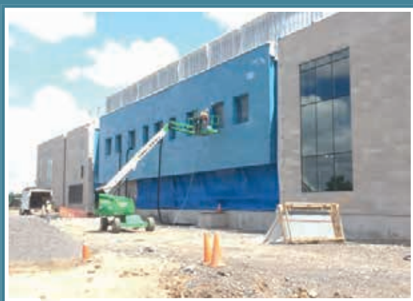
JUL. 10, 2017 Exterior metal wall work complete
